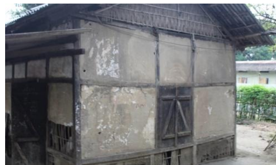
Fig 13 View of block beside entrance
