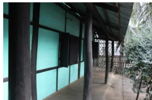
Fig.7 View of Veranda; Hajo Sal wood columns, mud flooring
