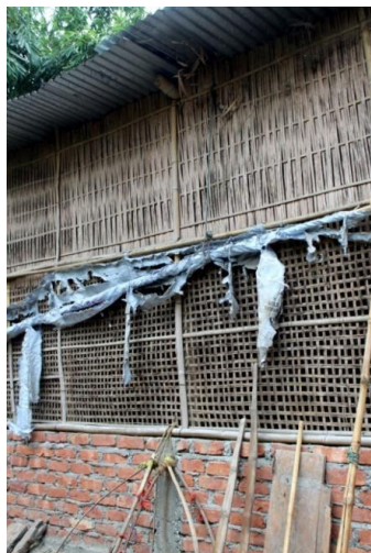
Fig 9 Posts to support spliced Bamboo wall
