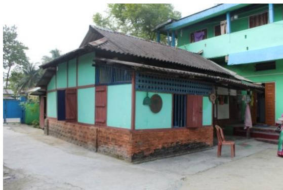
Fig 4. View of House 1
